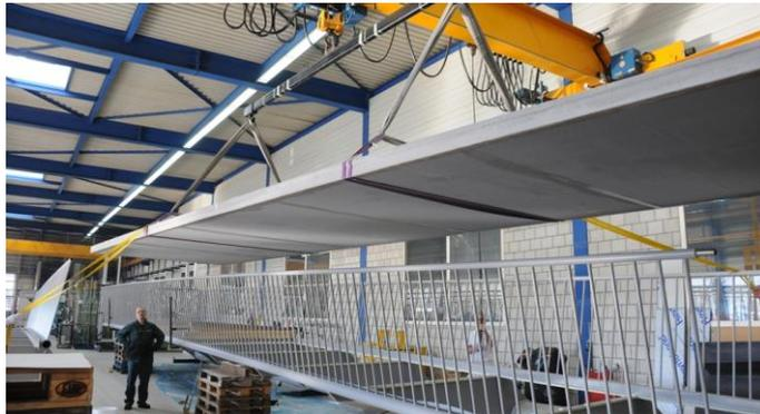
*Fig. 9 Composite deck element installation and adhesive bonding on steel substructure at metallic construction plant*
