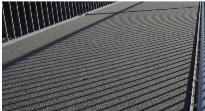
*Fig. 8 Composite deck with polymer concrete pavement, and composite flanges along both sides for water drainage*
