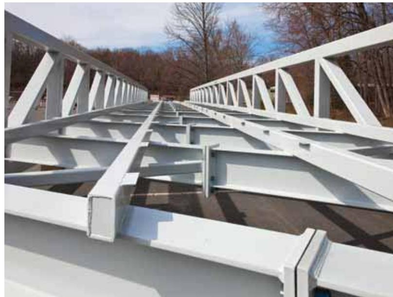
The superstructure of the Wolf Trap pedestrian bridge was a steel truss with longitudinal beams spaced 4.25 feet apart. Mechanical fasteners and Z clips provided the deck-to-beam connection.
