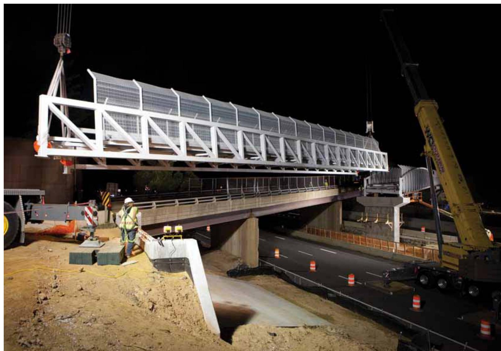
Nighttime construction has become commonplace to minimize the impact of lane and road closures. Composite Advantage supplied FRP bridge decks for a 3-span steel superstructure at Wolf Trap National Park. Here, the third span is lifted into place. The road was only closed for 15 minutes on three consecutive nights to accommodate the installation of each span.
